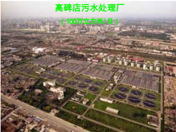
Fig-2 Gaobei Dian WWTP
