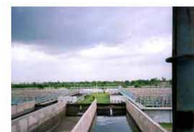
Figure 4: Sewage Treatment Plant Built By This Project
