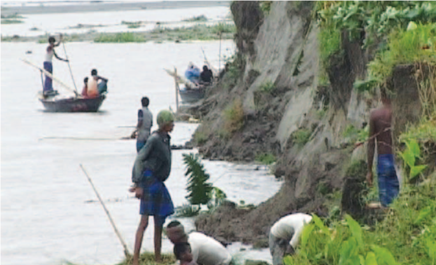
River Erosion (Source: PPA Field Study)
