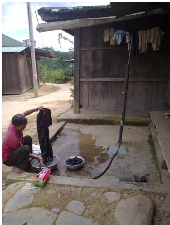
Water Pipe in Ta Vang Village: This pipe serves for 32 households in the village
