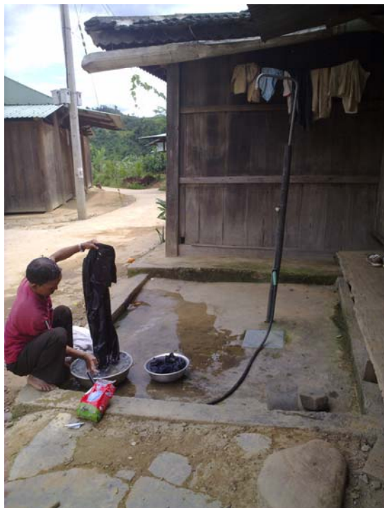
Water Pipe in Ta Vang Village: This pipe serves for 32 households in the village
