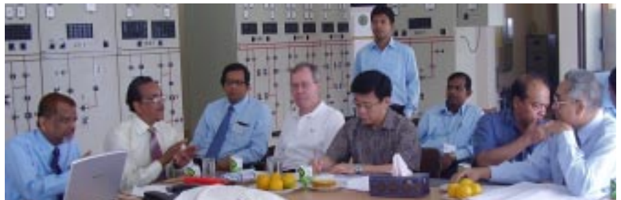
MEASURING PROGRESS Government officials brief SARD DG Kunio Senga (fifth from left) about work progress as he visits the ADB-assisted Amin Bazar power substation project
