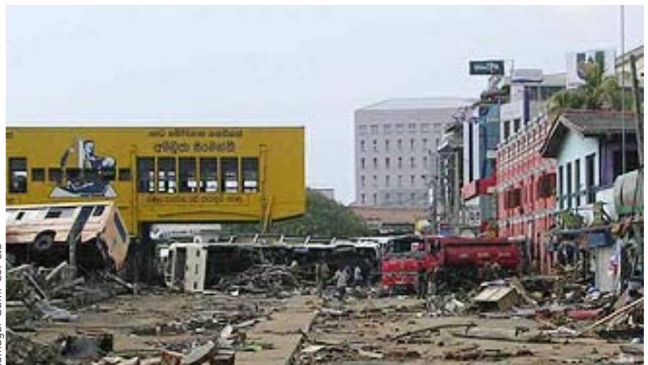
TSUNAMI DAMAGE Ruined Galle bus terminal in Sri Lanka
