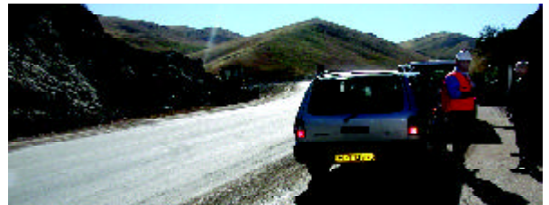
FIELD VISIT Hasan Masood, Senior Transport Specialist (left) discusses the state of the road with a representative of the contractor for civil works
