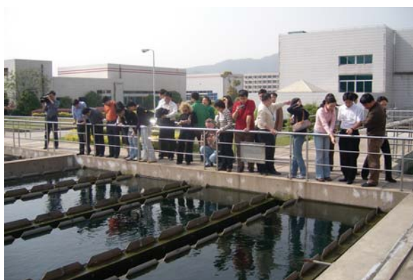
The program included a 2-day field trip, including this water sanitation facility in Huangzhou
