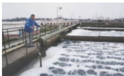
Anhui Environmental Improvement Project - A technician checking water quality at the Hefei chemical plant 安徽环保项目 -- 技术员检测合肥化工厂的水质
