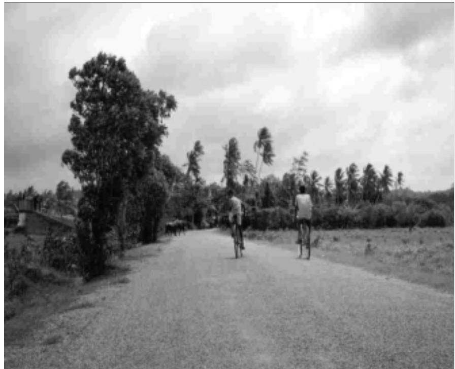
A rehabilitated road in Southern Province
