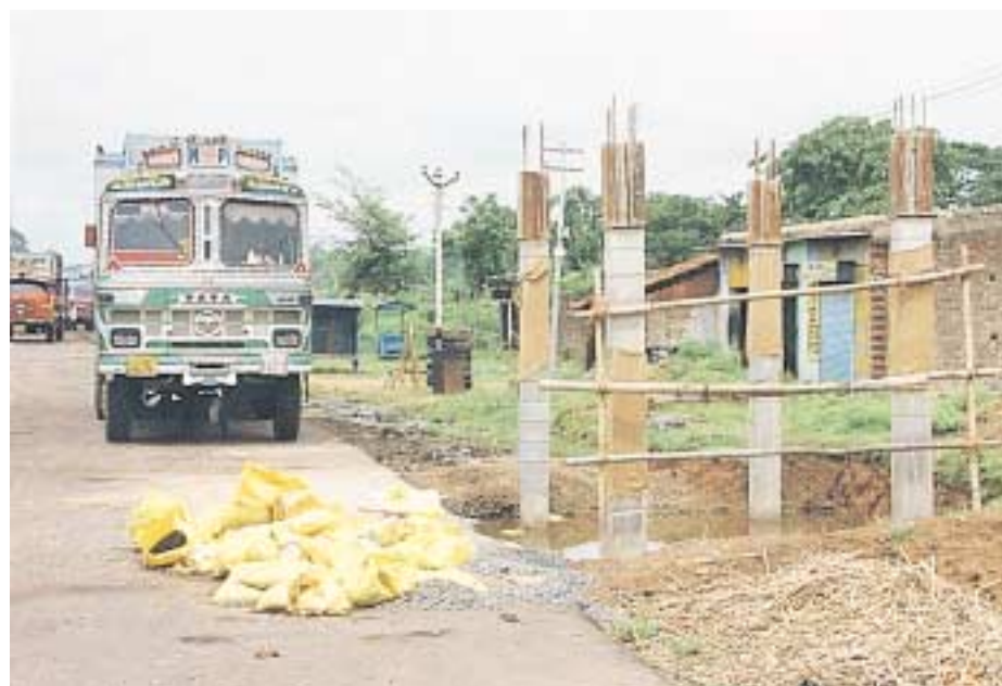
A bus shelter under construction on an Indian highway
