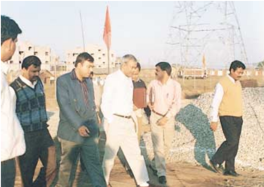
Power Grid and ADB officials inspecting progress at an ADB-assisted project site
