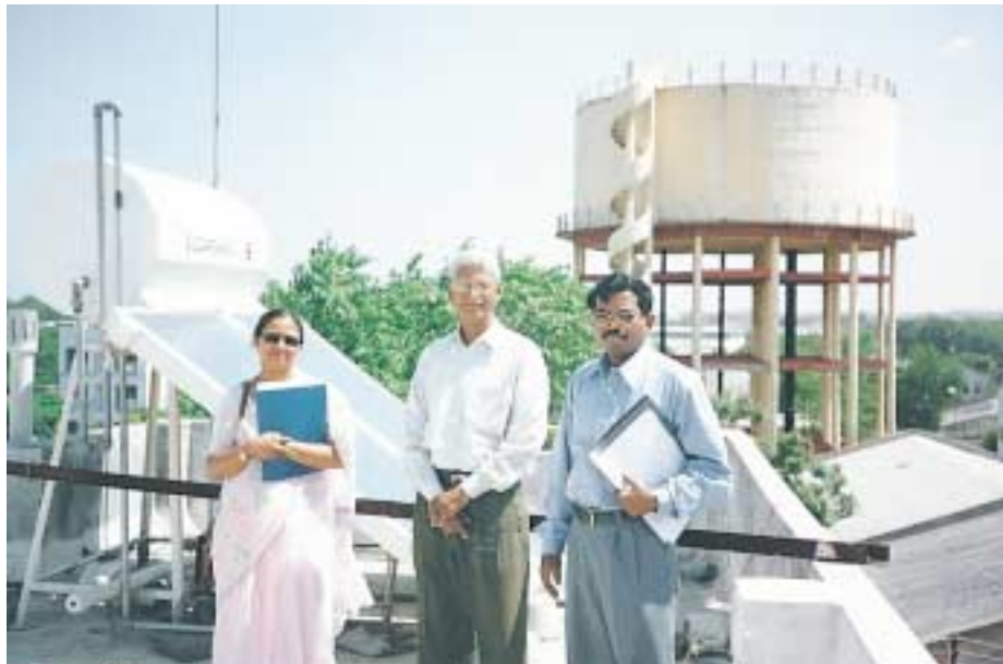
A solar thermal installation assisted under an ADB project
