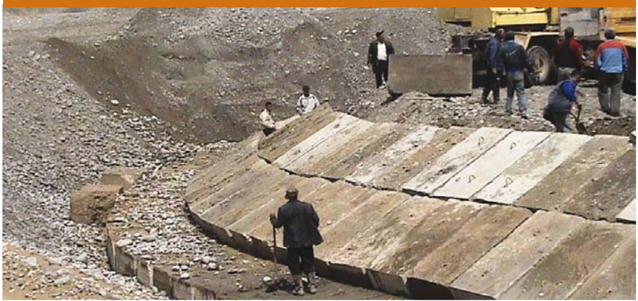
ADB is funding a flood risk management system in Khatlon, Tajikistan
