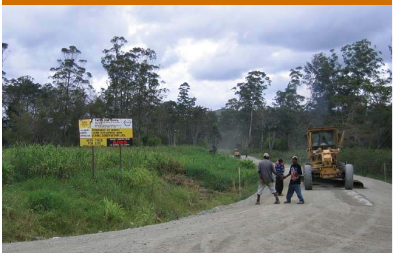
Roads are being upgraded in Papua New Guinea
