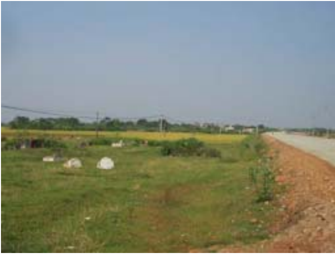
Near Phuc Yen Town. Completed section of the Expressway that avoided moving tombs.
