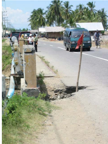
Kr. Bieng - Bridge to be widened
