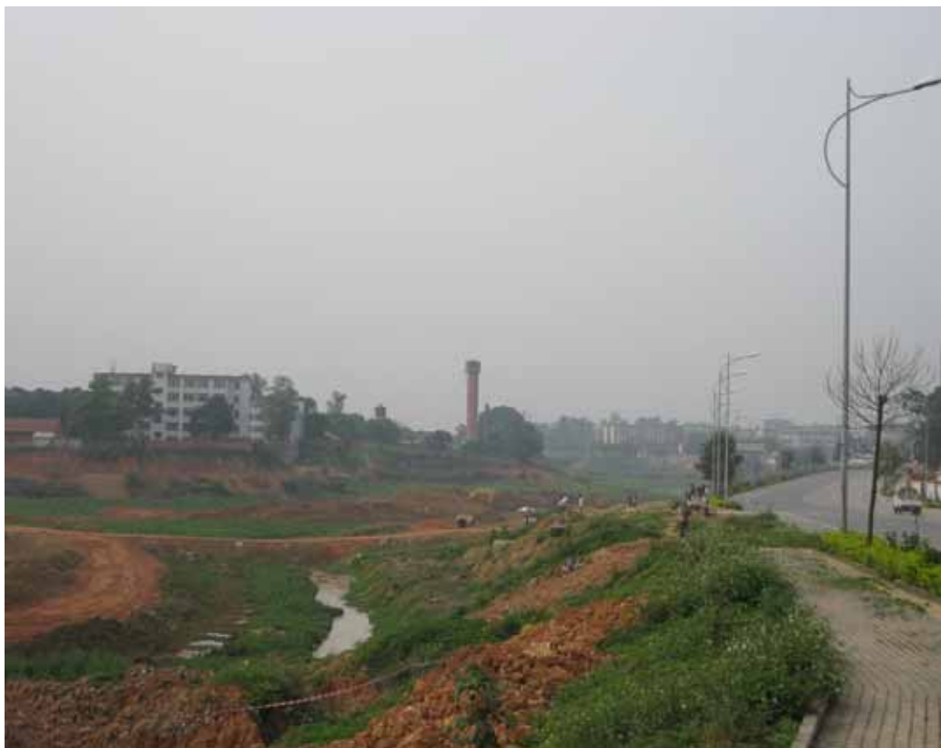
Figure 2-2 A Construction Site of Kelijiang Project
