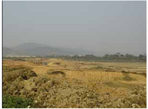
Works in progress on watercourse
