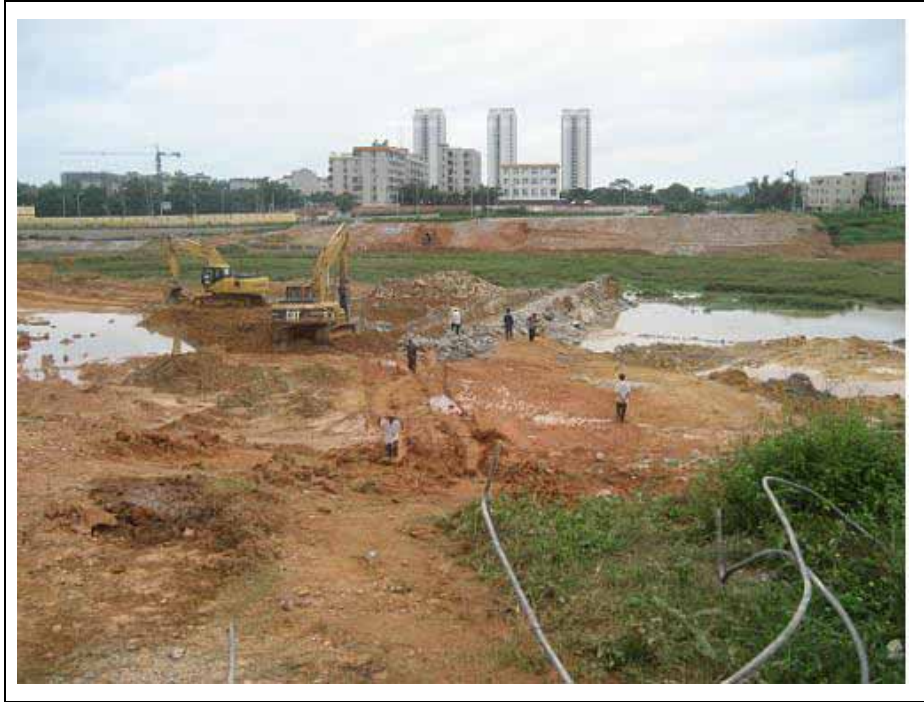
Picture 1-2 Construction site of bidding package
