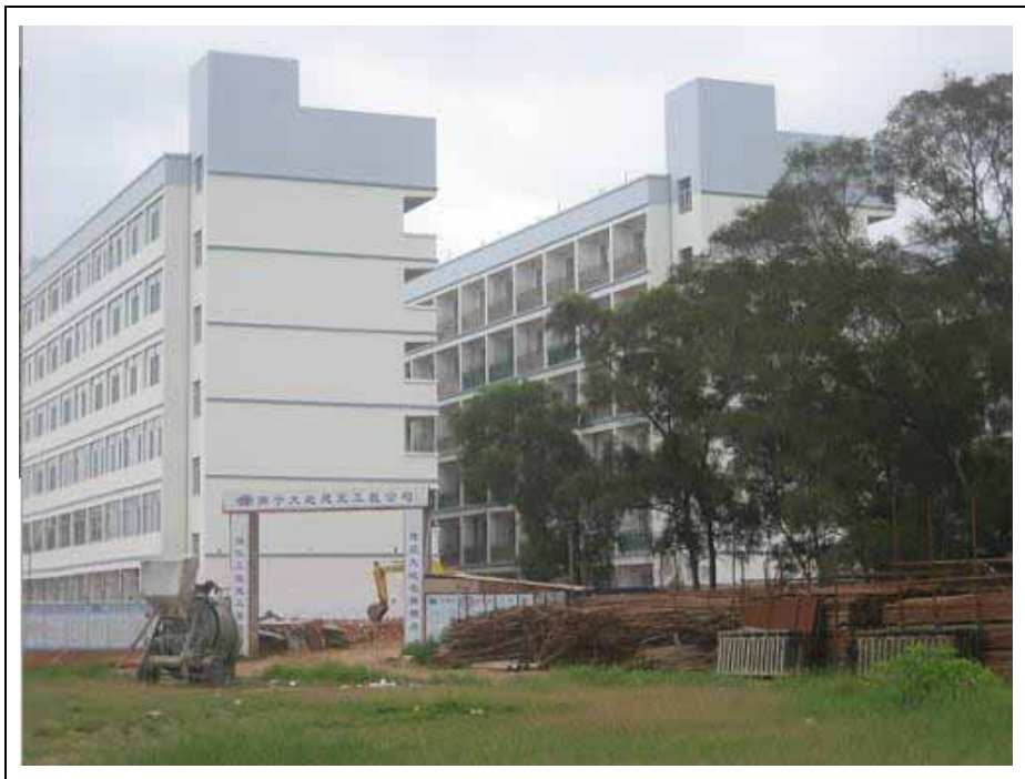
Picture 3-3 The newly-built students' dormitory buildings
