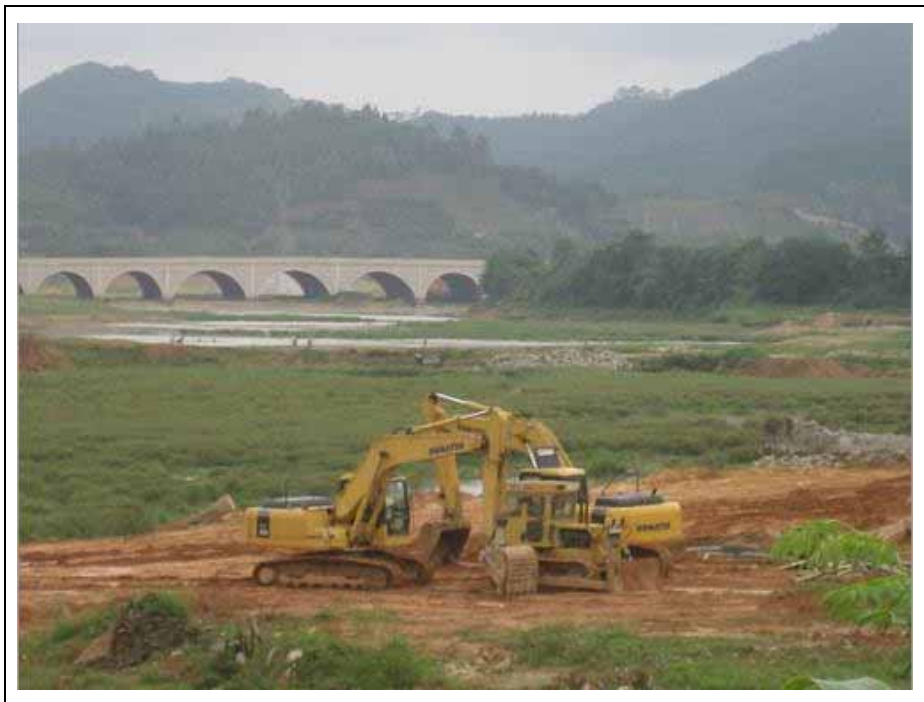
Picture 1-3 Construction site of bidding package
