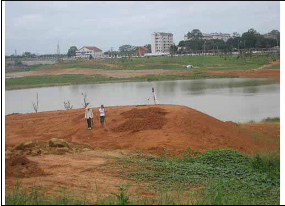
Picture 1-1 Construction site of bidding package
