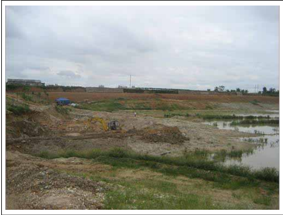
Picture 1-4 Construction site of bidding package
