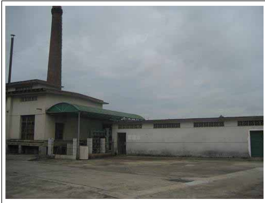
Picture 3-1 The affected old food processing plant
