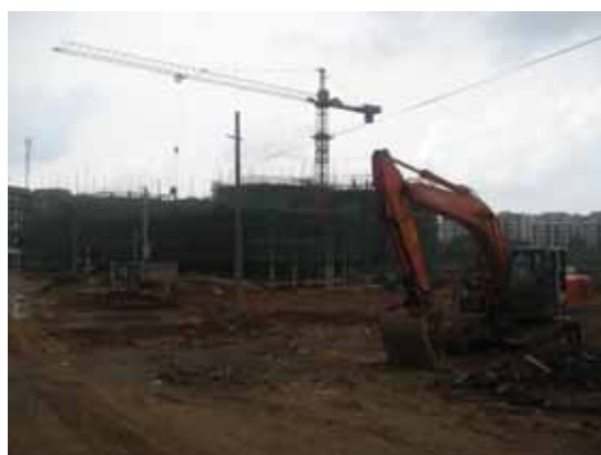
Picture 1-2 Two Buildings Being Under Construction in Xixiangtang Resettlement Residential Community
