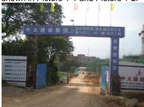
Picture 1-1 Xixiangtang Resettlement Residential Community Being under Construction
