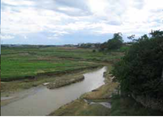
Picture 1-4 Construction Site of Xinxujiang Watercourse Treatment (South of Daxue Road)
