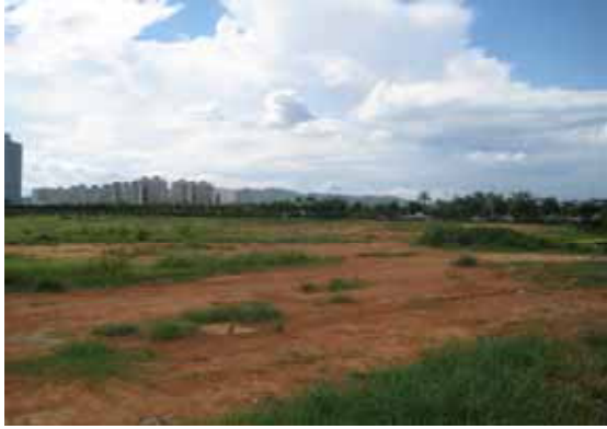
Picture 1-3 Construction Site of Xinxujiang Watercourse Treatment (North of Daxue Road)
