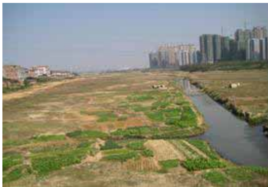
Figure 1-1 Construction Site of Xinxujiang Watercourse Treatment (North Daxue Road)
