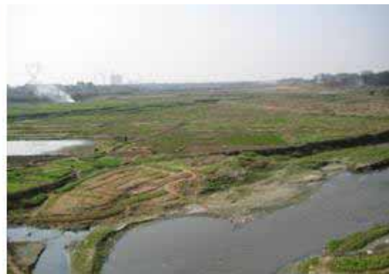
Figure 1-2 Construction Site of Xinxujiang Watercourse Treatment (South Daxue Road)
