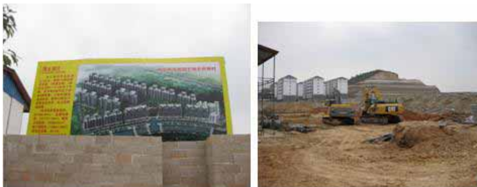
Picture 1-2 Fengling New Village under construction
