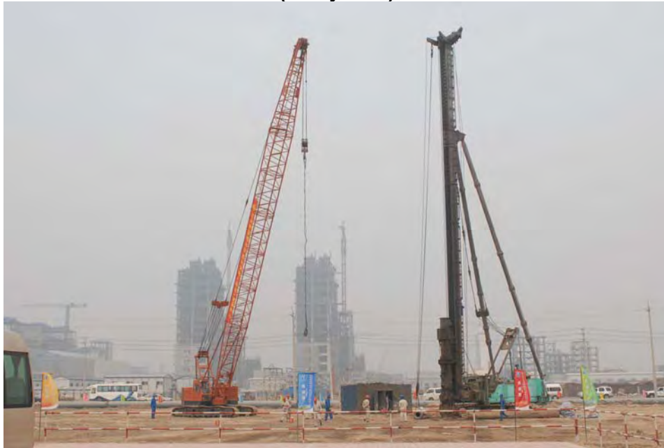
Figure A3.4: Foundation Treatment of Power Generation Island (6 July 2009)
