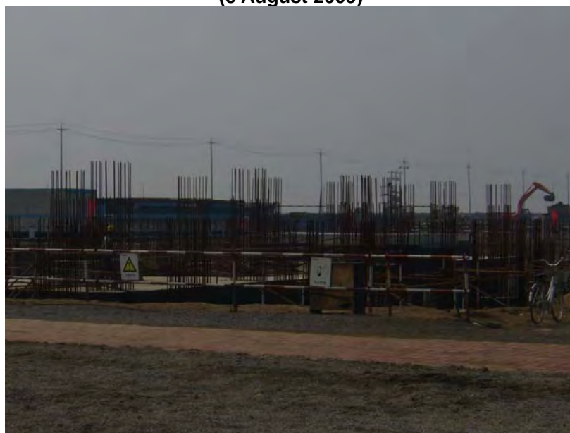
Figure A3.6: Construction Site of Air Separation Component (3 August 2009)
