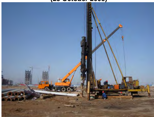
Figure A3.2: Ground Treatment of Project Site (25 October 2008)
