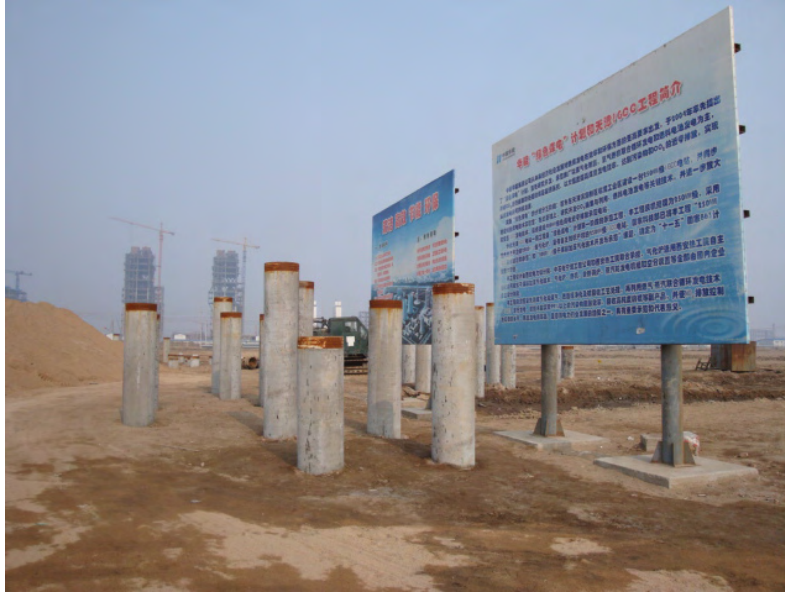
Figure A3.3: Foundation Construction of Coal Gasification Island (2 April 2009)
