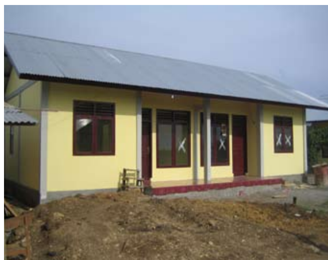
ADB-financed housing in Banda Aceh
