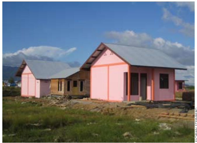
ADB-financed housing in Banda Aceh
