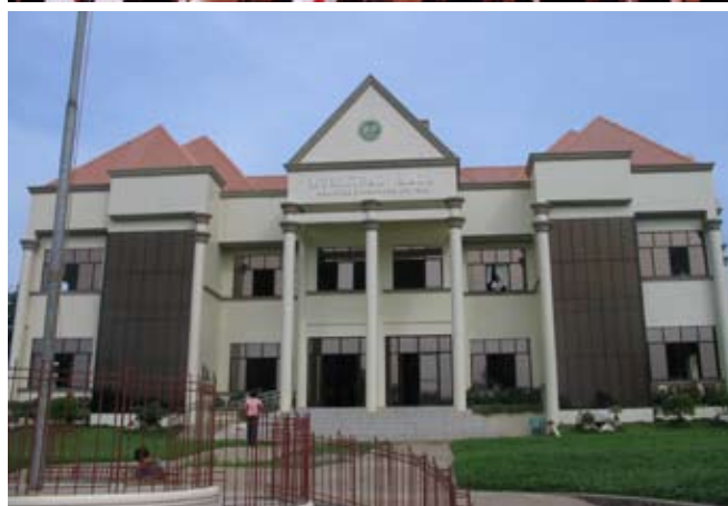
Mati public market (top) in Davao del Sur and the Mahayag municipal hall (above) in Zamboanga del Norte
