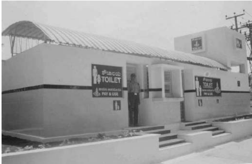
Figure 2. Community Toilets constructed under NIRANTARA
