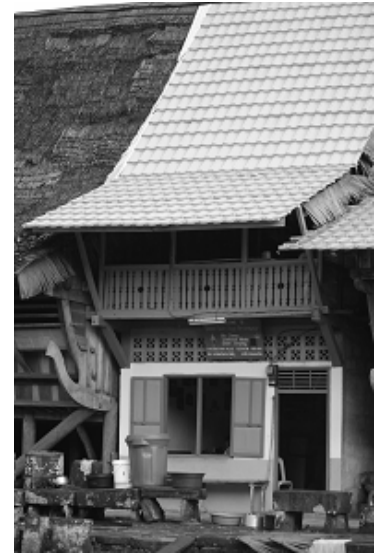
Rehabilitated traditional house without diagonal beam
