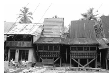
Rehabilitated traditional house with diagonal beam
