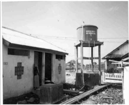
Water terminals operate in areas unconnected to network pipeline.
