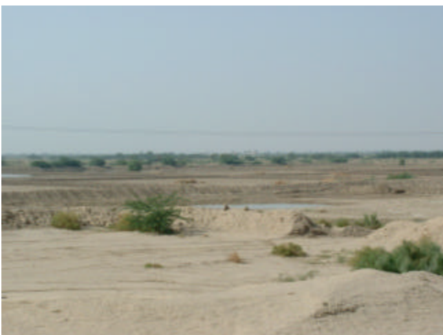
Rod Kohi embankment and retained water (near RD595)
