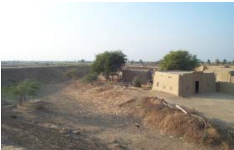
The wall around Katehrawali village
