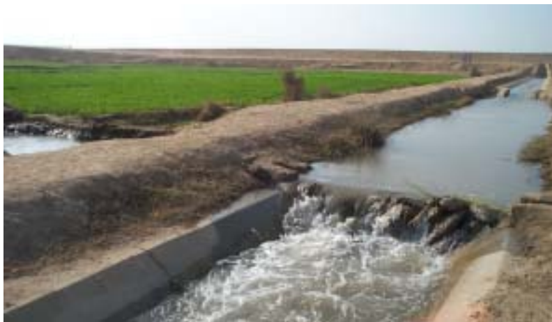
Distributary channel blocked to raise water to level of smaller channels.
