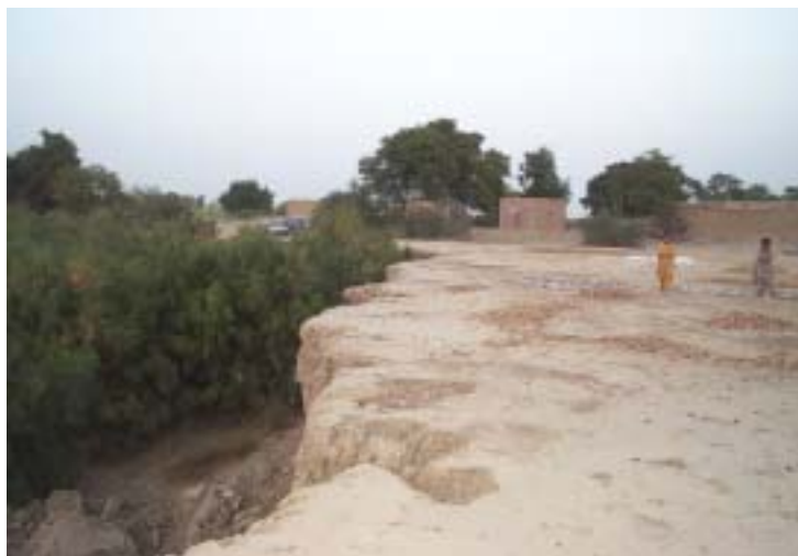
Erosion at Gat village
