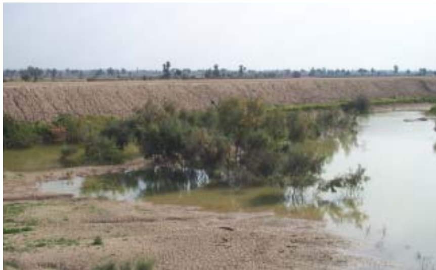
Ponded water on the west side of the canal
