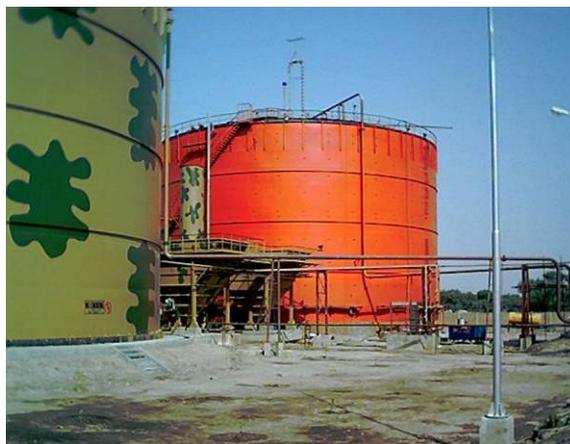
Wastewater treatment plant at Century Paper Mills along the National Highway near Pattoki, Punjab. This dissolved air flotation plant brings waste lint to the surface for capture and reuse.
