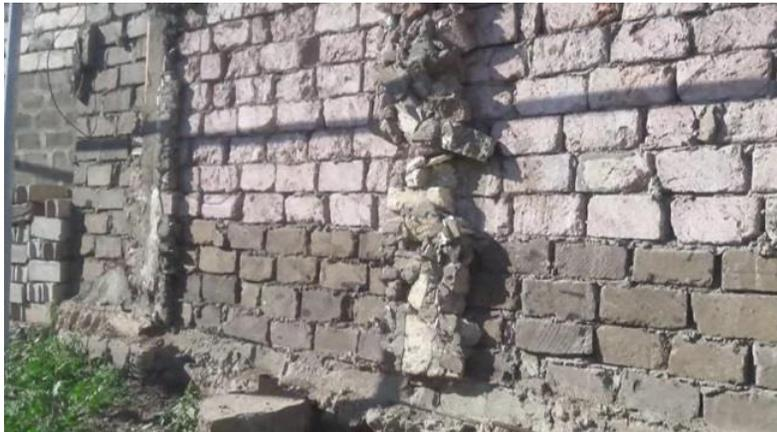
This wall used to be an "internal" wall but is now external and causes rain water seeping into the house.
