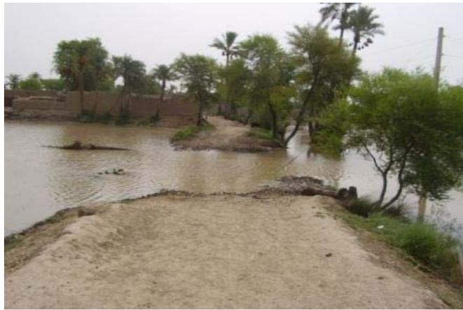
The embankment on the east of the village broken due to high floods in 1993-94 (main reason for the flooding)
