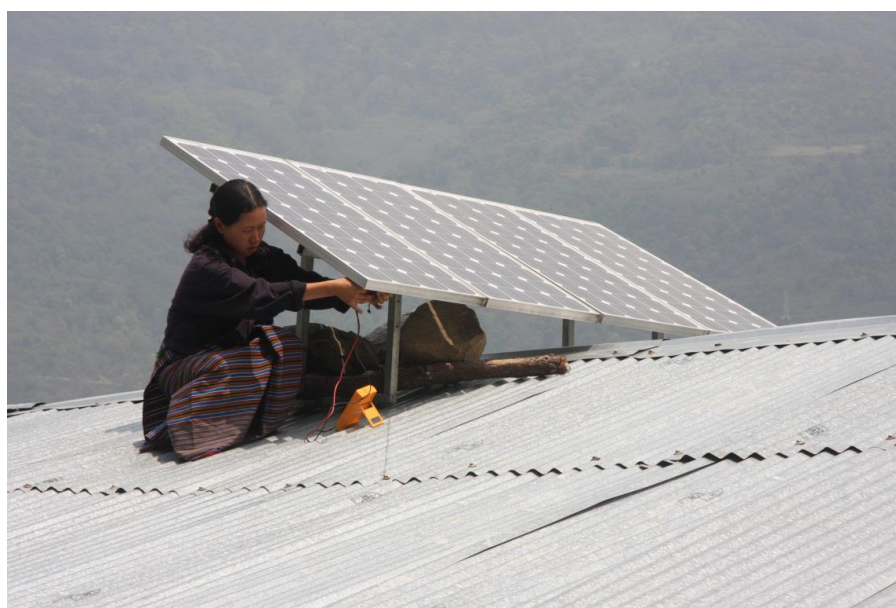
Local woman in Bhutan trained on the maintenance of solar photovoltaic panels.
