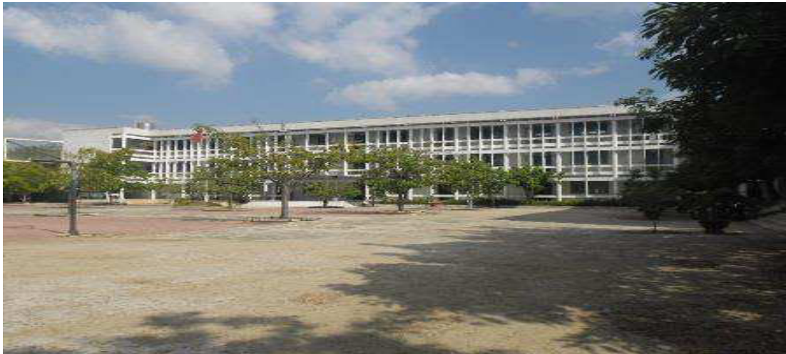
Front view of Ninh Hai Upper Secondary School.
