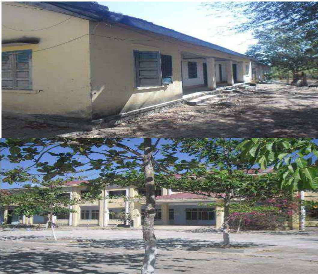
Existing buildings of the school.
