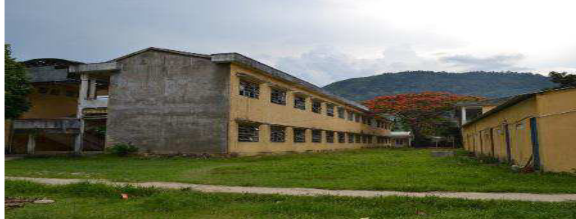
Existing buildings of Kham Duc USS.
