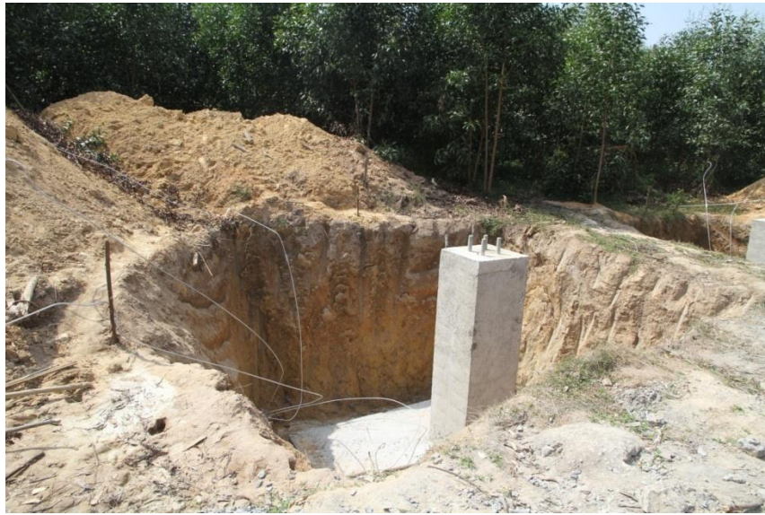
Figure 14-1 Foundation of tower under construction in Bac Tan Uyen
