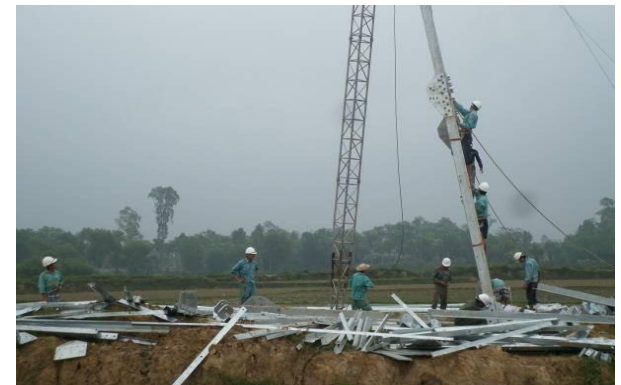
Photos 6: Workers wear labour protective clothing during tower erection
