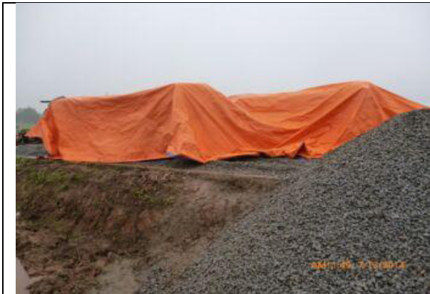
Photos 1: Worker is covering the material
