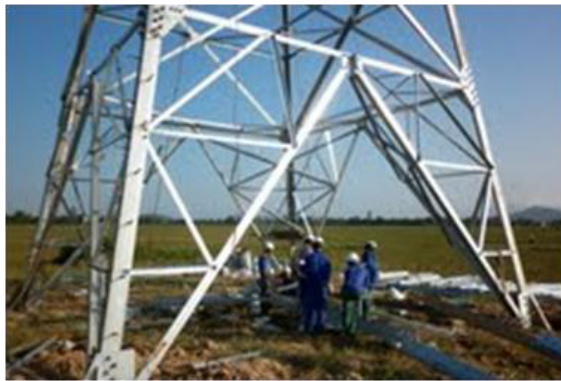
Photos 4: Worker is covering the material
