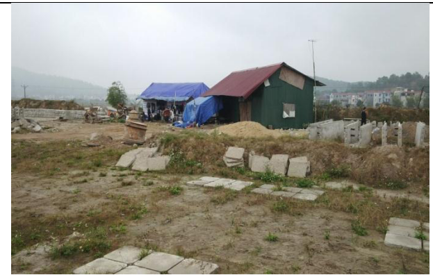
Photos 3: Temporary camps
