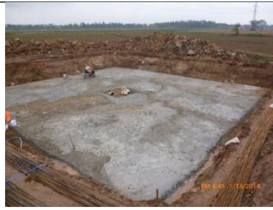
Photos 2: Consolidation by excavation
