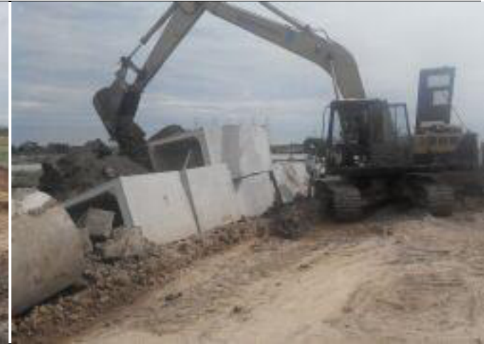
Photos 3: Traffic safety signs have not sufficiently arranged
