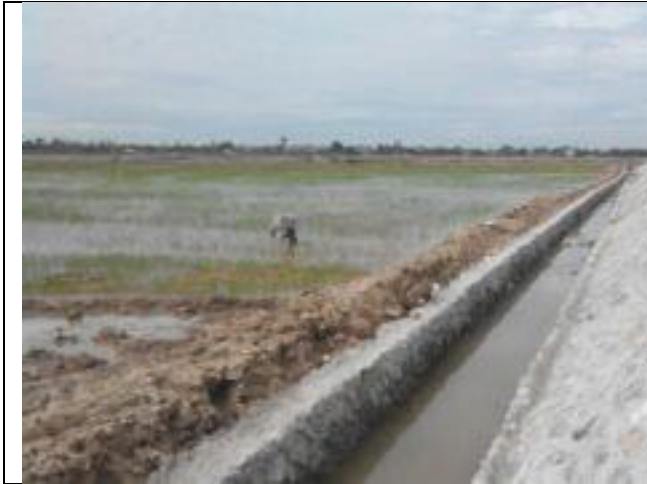
Photos 1: Stable foundation embankment at the access road to 500kV substation
