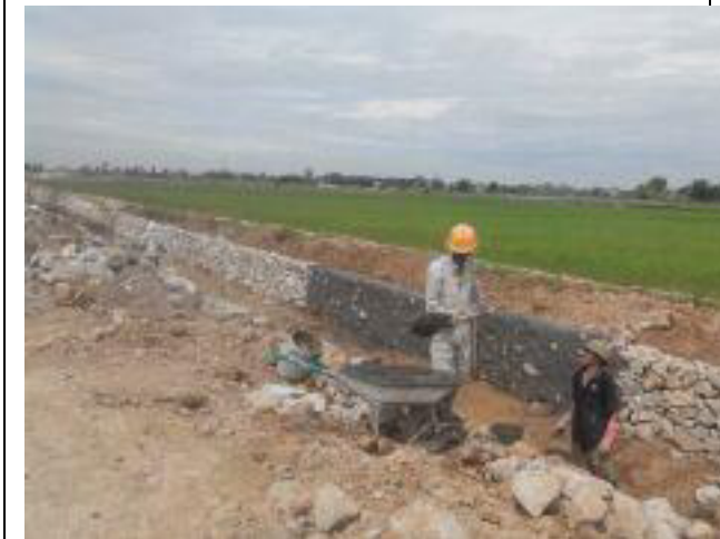
Photos 4: Worker is covering the material
