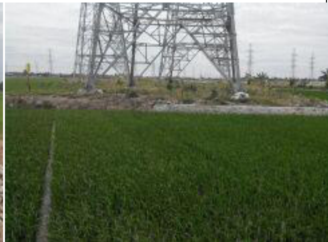
Photos 5: No waste found on the tower No19_220kV connecting line
