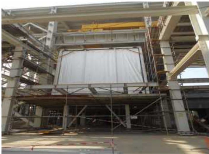
AIR INTAKE (LEFT) AND CONDENSER (RIGHT) ERECTION
