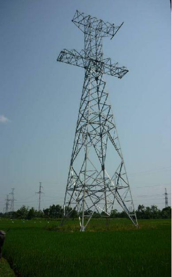
Photos 1: Tower was erected
