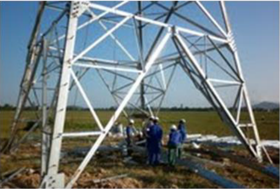
Photos 3: Workers wear labor protective clothing during tower erection
