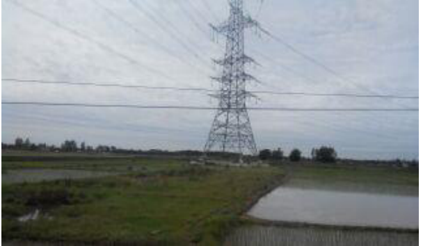
Photos 4: Civil work has almost accomplished
