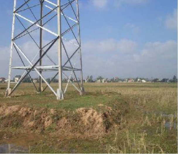
Photos 2: Rehabilitation upon completion of tower foundation
