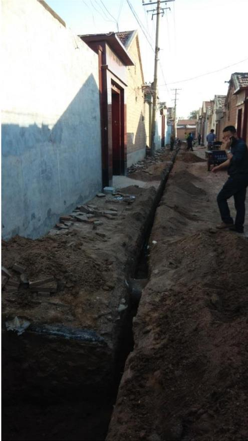
Picture 3: Ditch excavation in lane
