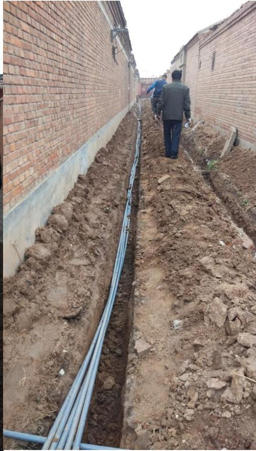
Picture 4: Pipeline laying in lane
