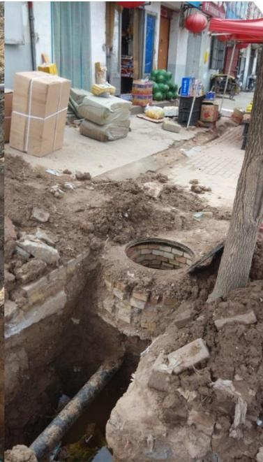
Picture 6: Road excavation and pipeline laying in downtown
