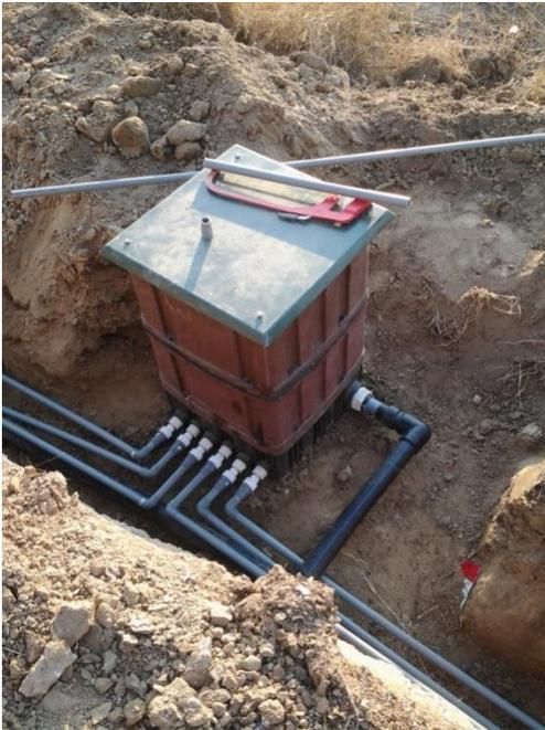
Picture 5: Water meter chamber excavation
