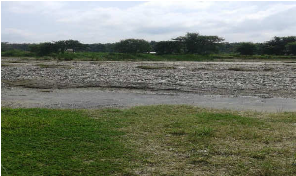
Figure 6 Luandra river crossing work
