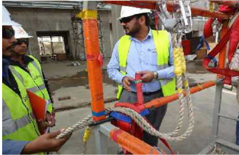
WEEKLY WALK THROUGH AND PPE INSPECTION
