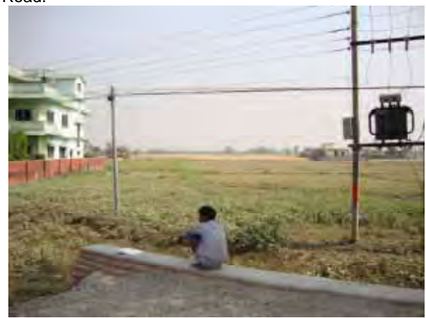
Km 0+140 onwards, the proposed road traverses along open cultivated field. Noted Transformer will require Relocation.
