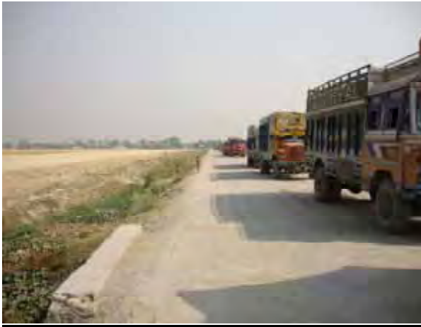
Bituminous Link Road leading to Sunauli Custom
