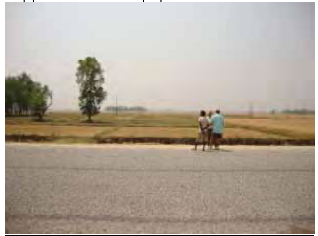
End point Junction at km 3+340 meeting Bhairahawa – Parasi Road.
