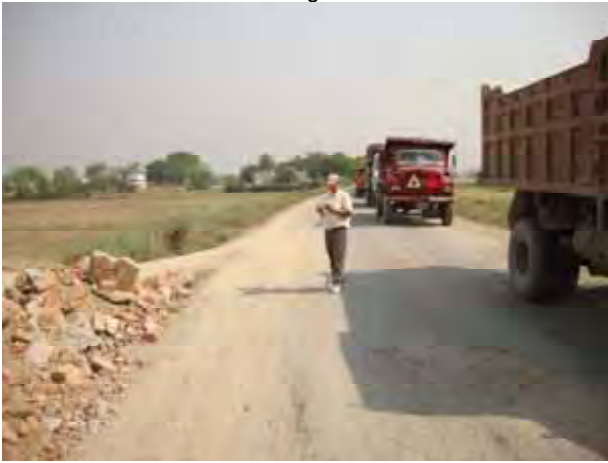
Starting point of Proposed Bhairahawa Bypass (BBY) Road
