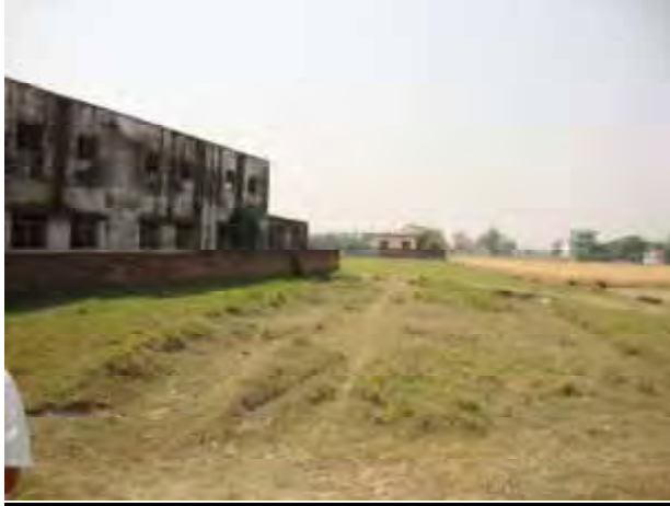
Km 0+420 viewing west, where built up compound wall structure lies near ROW.
