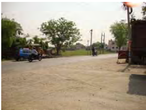
Junction at Km 0+130, where BBY road meets Bhairahawa – Sunauli Highway. Requires appropriate Junction Improvement.
