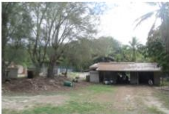
Existing power house in Mauke Island to be relocated to proposed solar power plant
