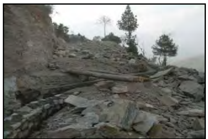
Rehabilitation of irrigation canal at Solukhumbu
