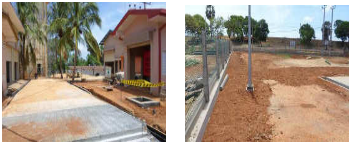
Figure 3.1. Site cleaning and landscaping works in progress at Murunkan site
