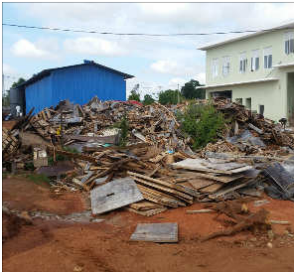
Figure 5.2. Construction debris collected to be removed – WTP at Vavuniya
