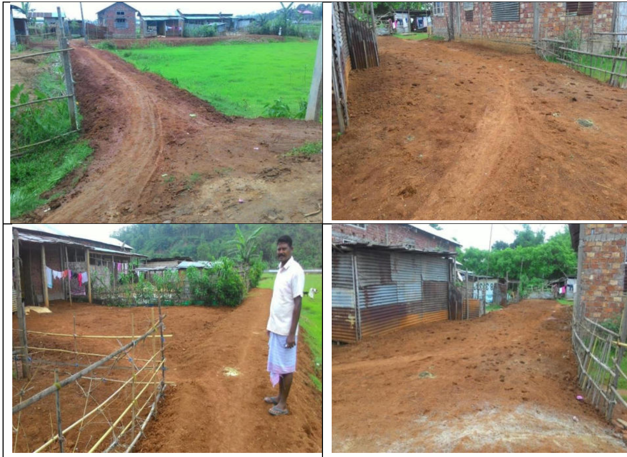
Figure 3: Photographs of Additional Land Filling at Kochpara Rehabilitation Site, Palashbari
