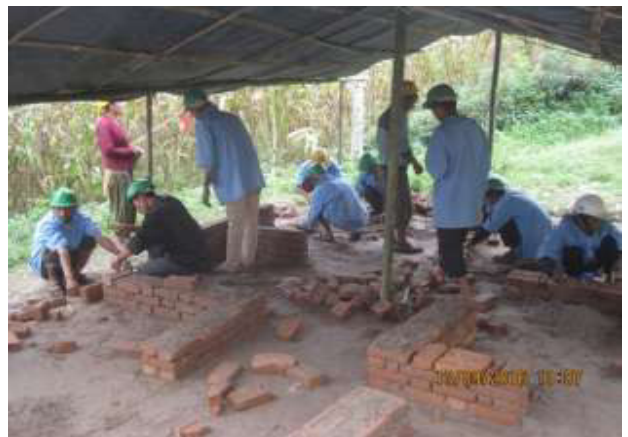
Practical work in brick layer mason training
